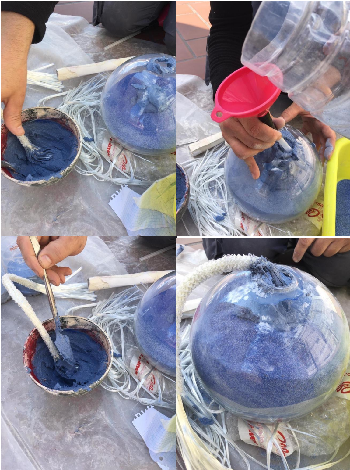
Fig.3-6: Application in Casa Batlló's roof ornaments. Use of carbon fibers and lime mortar to fix the decorative spheres on top of the roof chimneys. Carbon fibers that replace the previous iron rods, which on the outside and over the years, came to produce breakage of the original spheres. ©Joan Olona & Mireia Bosch
