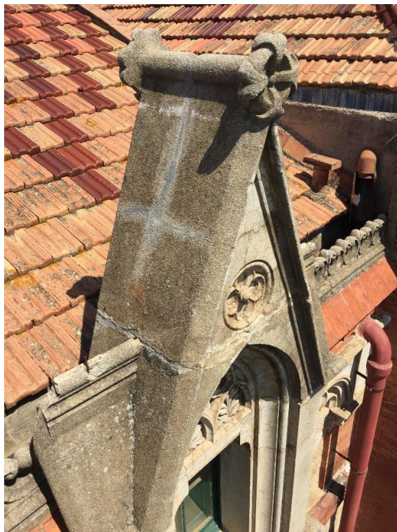
Fig.1-4: The images show the characteristic stone decorative elements of the buildings of the early 20th century, which show movements and cracks, since they are supported only by their own weight. ©Josep Baquer
