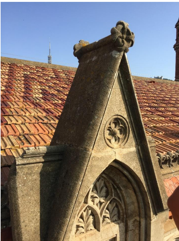
Fig.1-4: The images show the characteristic stone decorative elements of the buildings of the early 20th century, which show movements and cracks, since they are supported only by their own weight. ©Josep Baquer
