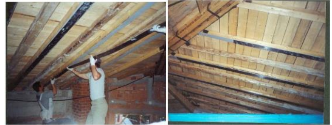
Fig.1: Renovation of wooden roof.
