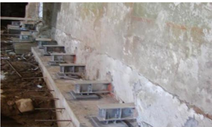
Fig.16: Extension of the foundation base, connection between the foundation and the reinforced concrete beam-curbs.
