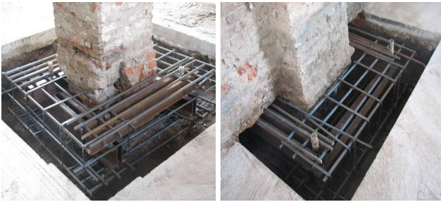
Fig.1-2: Execution of reinforced concrete curbs. Intervention carried out in the d'Este Castle of Arquà Polesine, Rovigo.
