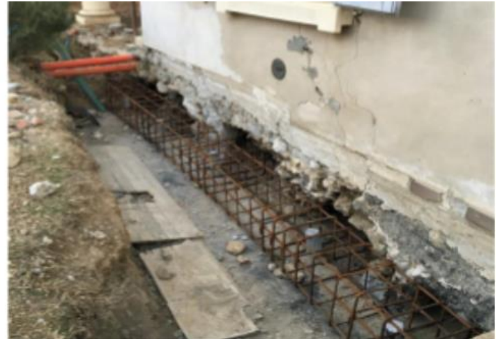
Fig.15: Extension of the foundation base, positioning of the reinforced concrete beam-curb.
