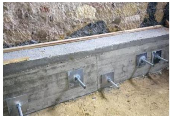
Fig.16: Extension of the foundation base, connection between the foundation and the reinforced concrete beam-curbs.
