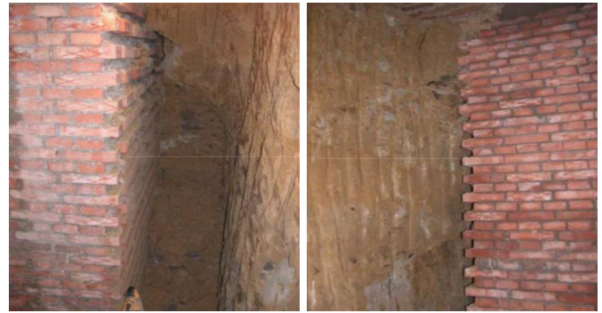
Fig.7-8: Intermediate phases of consolidation work.
