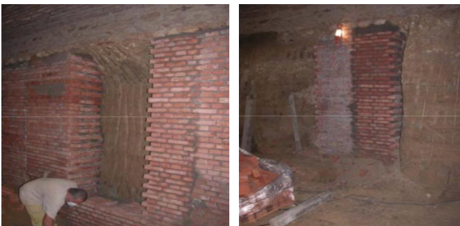
Fig.5-6: Realization of sub-building consolidation works.
