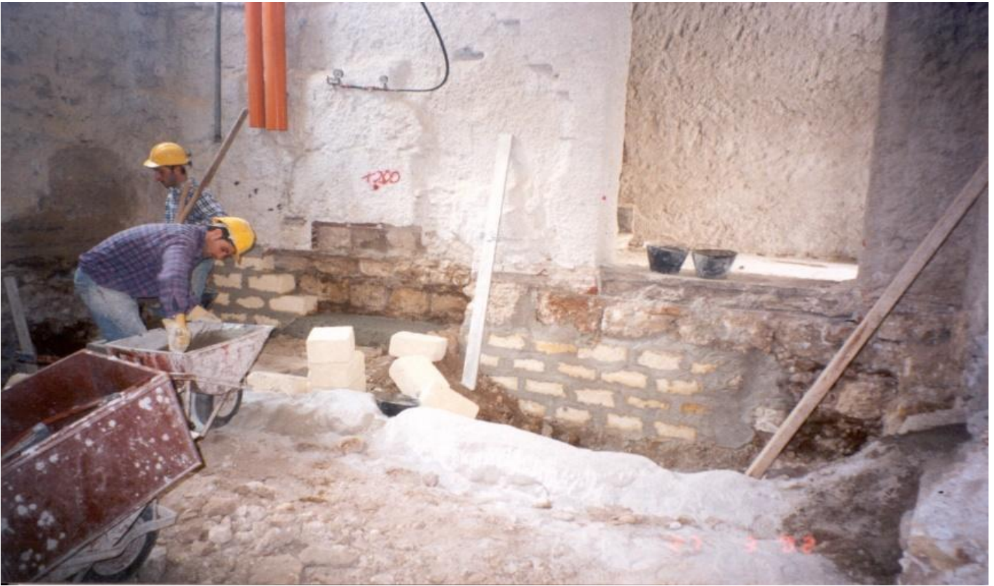
Fig.17: Masonry foundation consolidation. © Mario Li Castri
