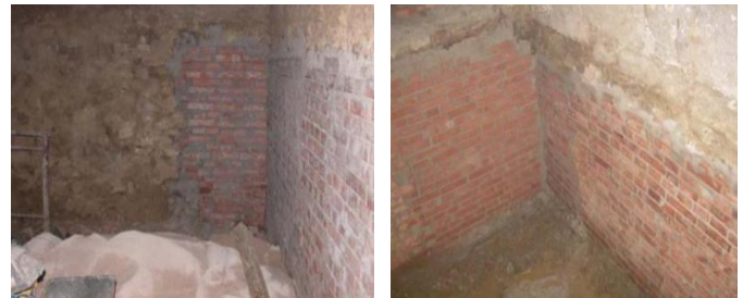
Fig.9-10: Final phase of consolidation work.
