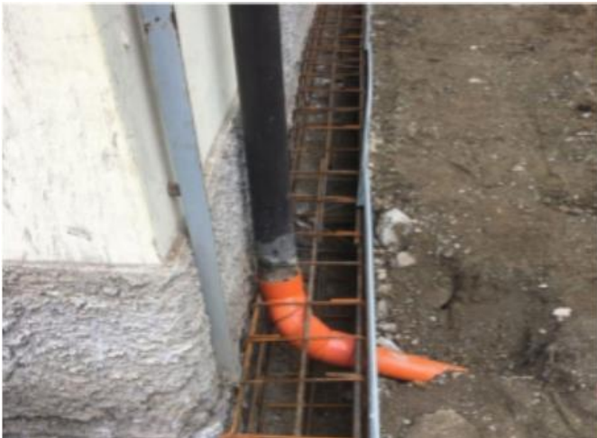
Fig.15: Extension of the foundation base, positioning of the reinforced concrete beam-curb.
