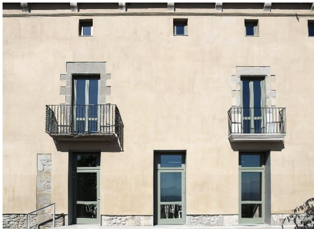
Fig.7: Rehabilitated wall in which a test campaign was carried out.
