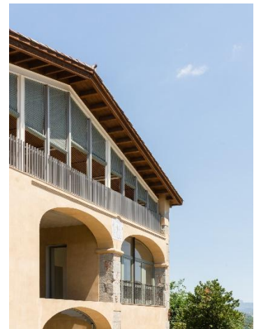
Fig.9: Façade of rammed earth and masonry, connected to interior walls with anchors.
