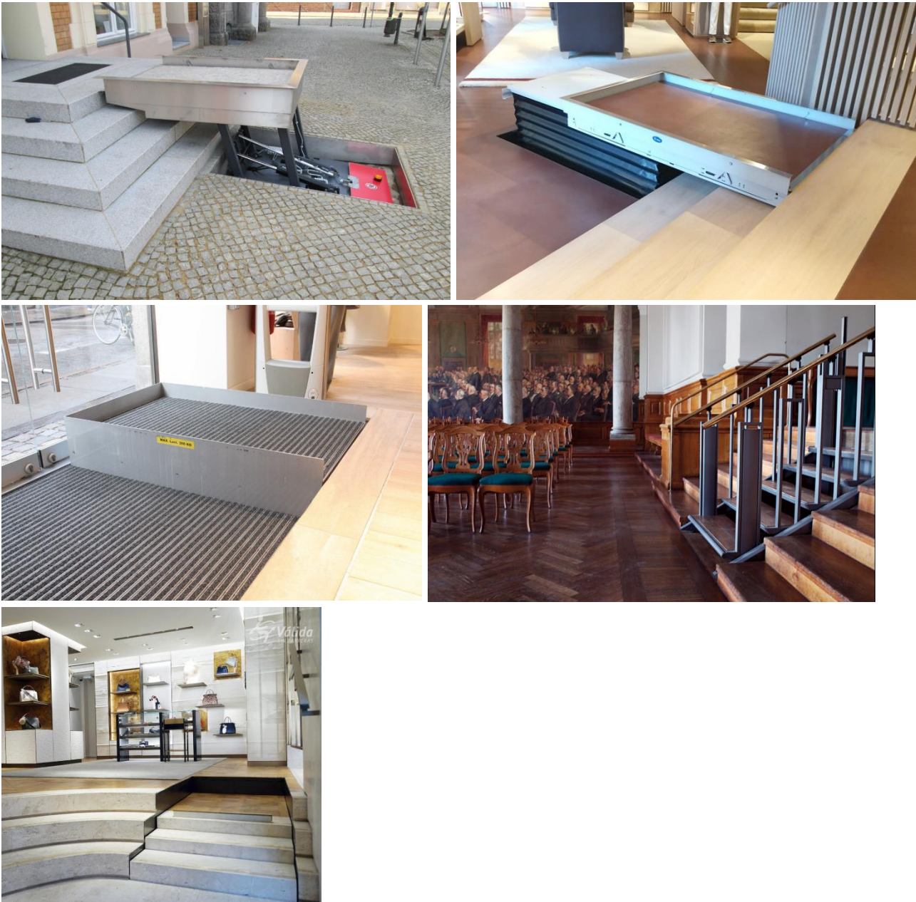
Fig.24-28: Examples of low-profile short-travel lifts, ideal for places where a discreet solution is needed. These models are intended to blend with the surrounding architecture and to not be noticed at first sight. It's a solution consisting of a platform lifted from below by a mechanism, and sometimes it includes railings, depending of each case. ©Váldasinbarreras
