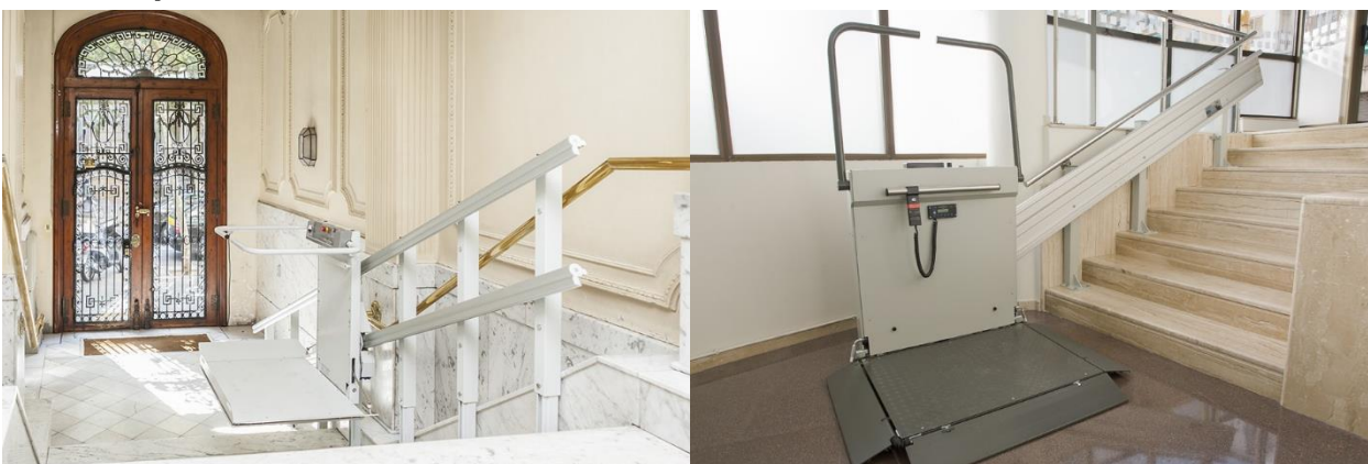
Fig.8-9: Examples of stairlift platforms, ideal for places where an elevator is not feasible and a difference of height, with steps in a straight-line path, is present. It relies on a rail attached to one side of the stairs, and a platform with security guards so people in wheelchairs can overcome the obstacle. This solution is generally used in halls with protected or catalogued stairs where a ramp is not permitted, or it doesn't have enough room to be installed in compliance with the required standards. ©Váldasinbarreras
