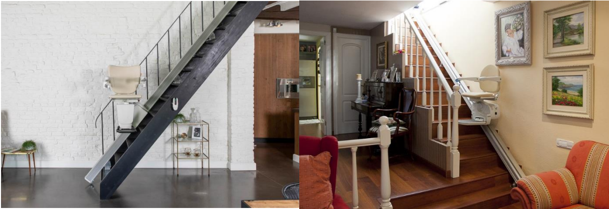
Fig.1-2: Examples of stairlift chairs used ideal for spaces where other solutions, like elevators, are not feasible. It relies on a single rail attached to one side of the stair, where a foldable chair is placed to run the length of said rail. This solution is intended for single flights of stairs with a straight-line path. ©Váldasinbarreras
